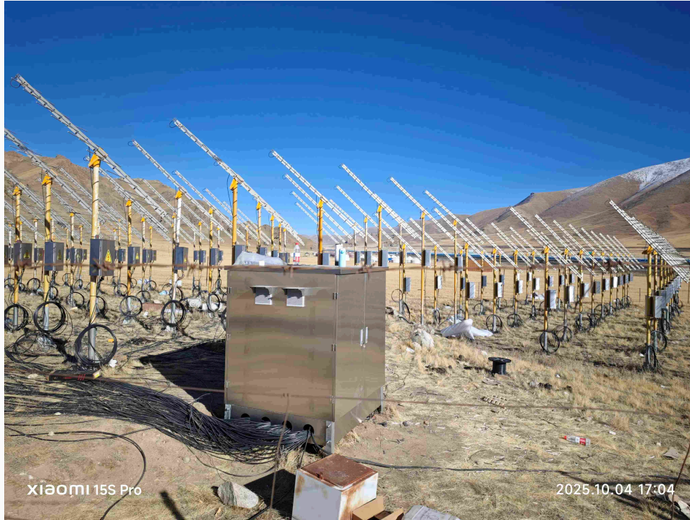
Figure 18: Two stations with remote-controlled signal delay tuners installed.
